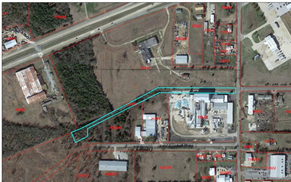
Rail Construction Services Site
